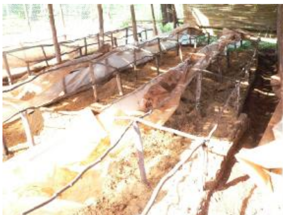
Figure 3: Banana macropropagation structures can be constructed on a low budget using affordable and locally available materials.
